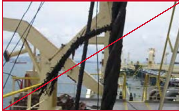
Lifeboat wire that will not pass inspection.
