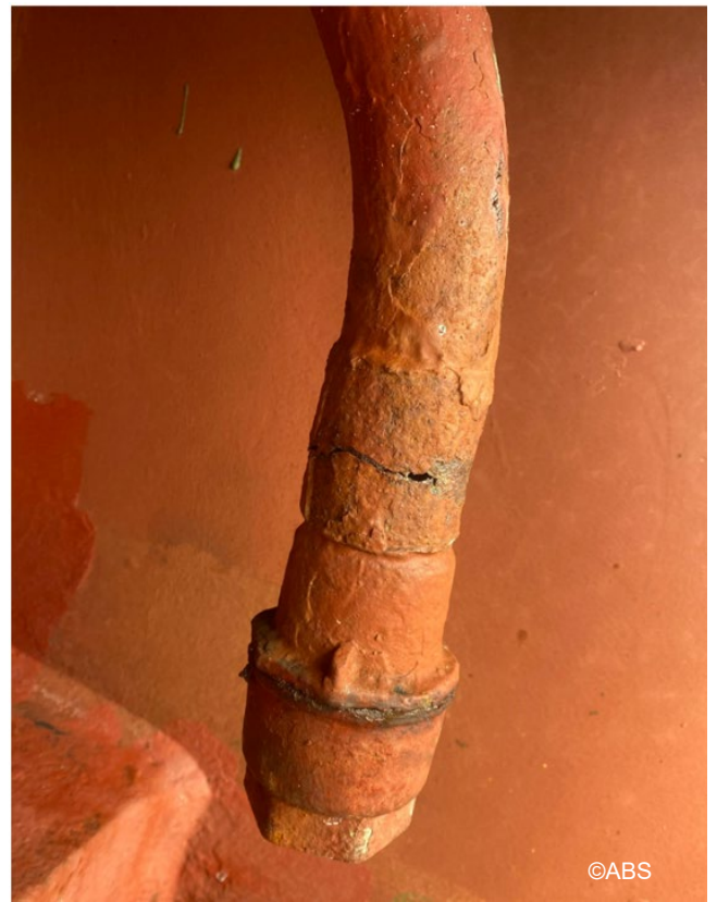
Drainpipe for hatch coaming found with rust and hole
