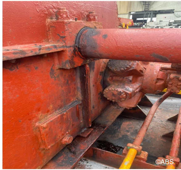
Oil leakage from winches on deck
