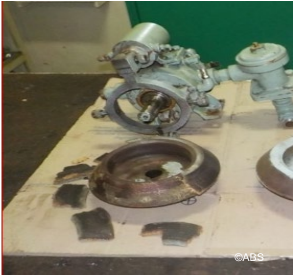
Clutch for vacuum unit of emergency fire pump broken
